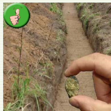
Pic. 2 Sandy compact trench bottom
