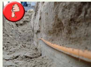
Pic. 1 Duraflat copying trench bottom
